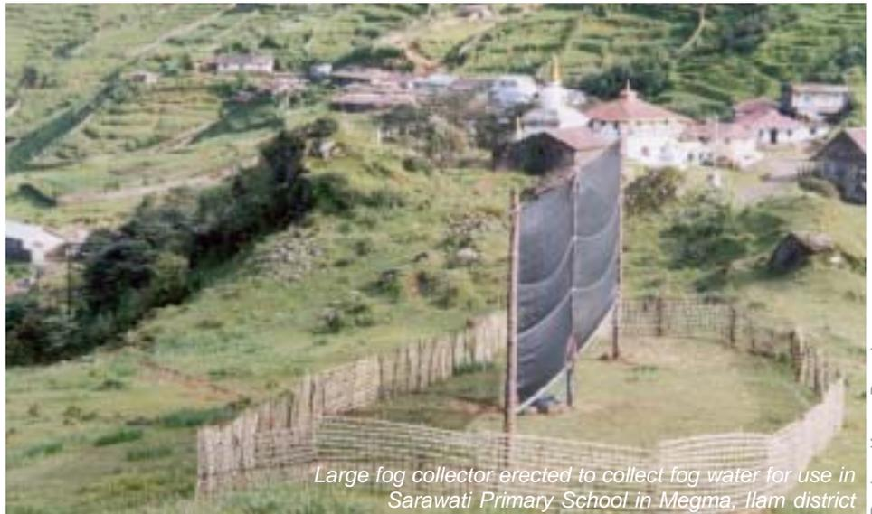
*Large fog collector erected to collect fog water for use in Sarawati Primary School in Megma, Ilam district*
