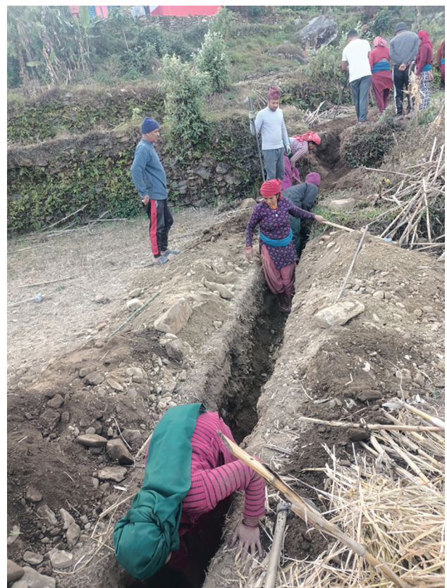
Pipeline digging work at Kavredanda Lift WASH Project, Baglung Municipality-13
