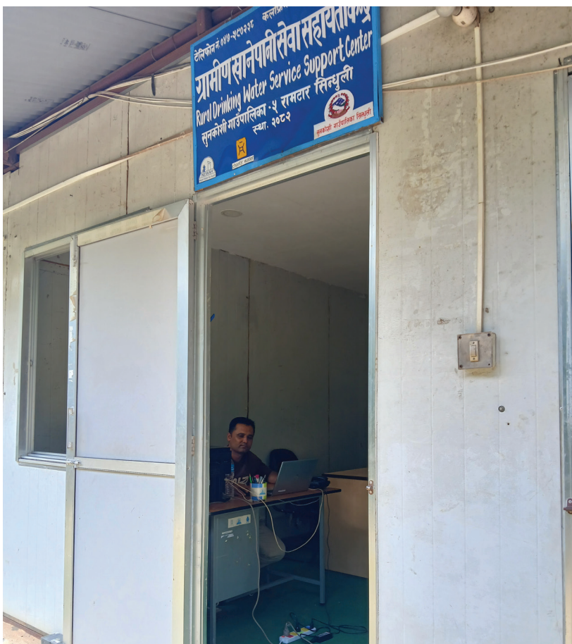
Service Support Center established in Sindhuli
