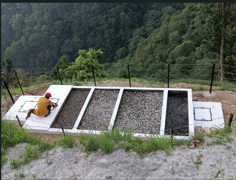
Horizontal Roughing Filter
